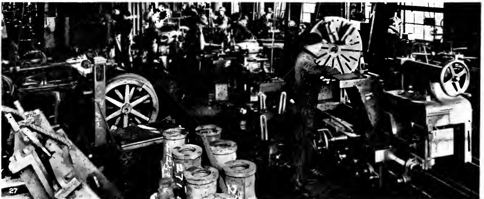
The shop of the Harris Ice Machine Company, Portland, Oregon, where a large business in refrigerating machinery has been developed.
